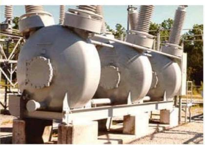
Three phase transformers are used throughout industry to change values of three phase voltage and current. Three phase power is the most common way in which power is produced.
